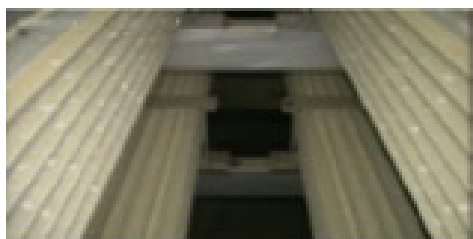
Figure 9: Salt can be seen forming on the aluminium extrusion. These extrusions are shown supported and strapped to the structural stainless-steel box-section
